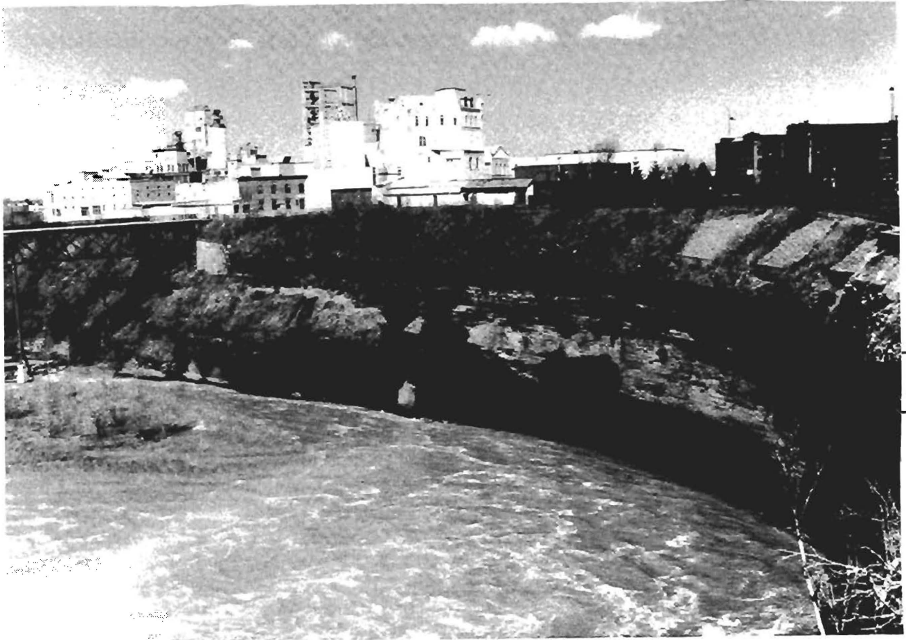
FIGURE 24 East side of gorge below Upper Falls. Genesee Brewery in center and left of photo. Rock Units: 1=Lewiston Mbr.-Rochester, 2=Gates Mbr.-Rochester, 3=Decew Fm. (Bill Clar)
