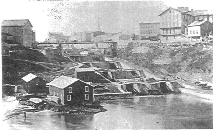
Figure 13 Lockport flight of combined locks, circa 1880. Note canal boats in lowest and uppermost chambers of the west flight. Rochester Shale capped by Decew Dolostone on right (west) bank.
