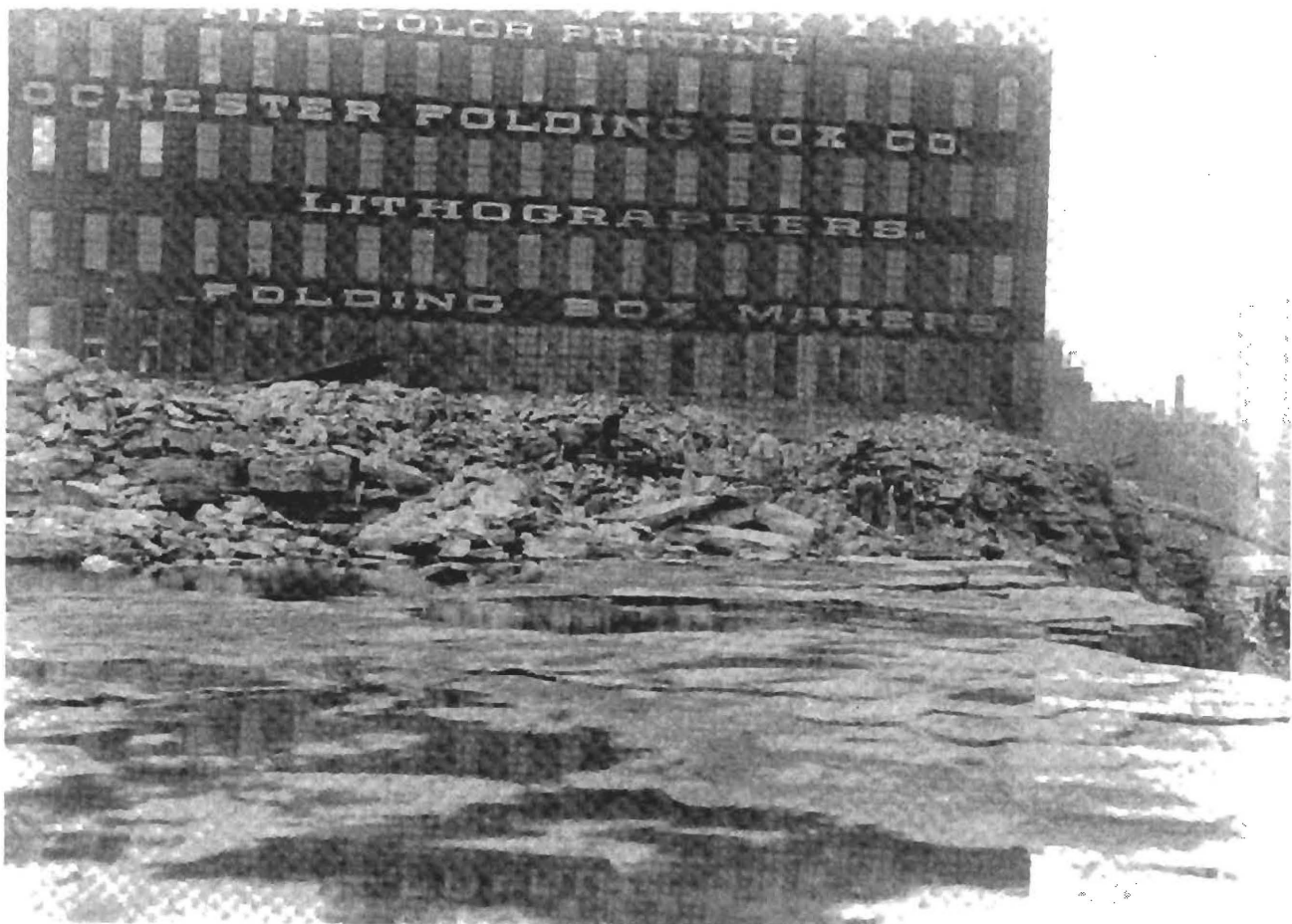
FIGURE 26 High Falls showing rock debris from blasting. Looking west. Gorsline Building in distance. Nov. 1914. (Stone Collection, Roch. Mus. and Sci. Center)
